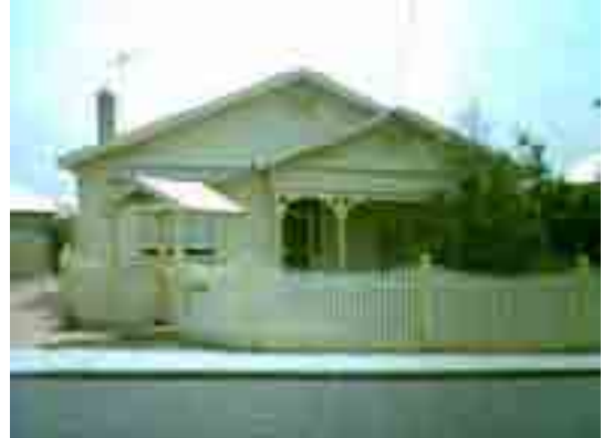
2009: Interwar Bungalow, Elizabeth Street, with altered verandah fretwork & single posts.
