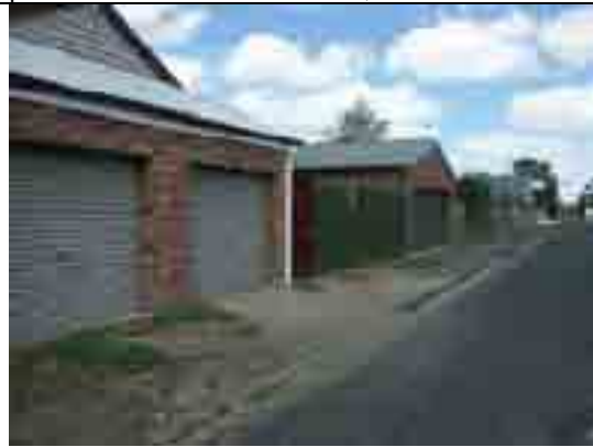
Photo 7.12: Rear garages fronting onto Potter Street. Source: David Rowe, 2008.
