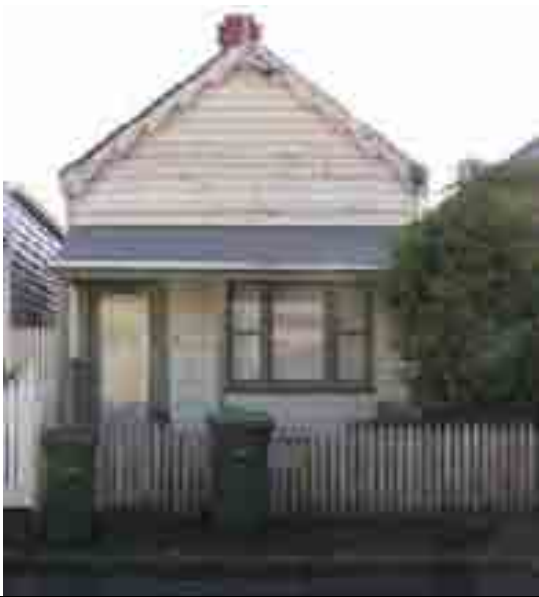
Photo 10.19: Residence, 14 Weller Street. Source: City of Greater Geelong, 2008.
