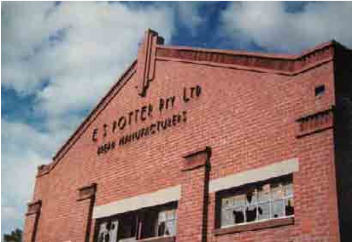
Figure 9.32: Potter Bakery (Lupton Street façade), 1986. Source: Aitken, Honman & Huddle, 'City of Geelong West Urban Conservation Study', 1986.
