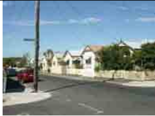
Photo 6.06: Homogenous streetscape of Edwardian dwellings at 13-27 George Street. Source: David Rowe, 2009.
