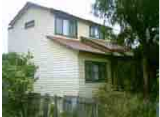
2009: Altered Edwardian dwelling with large 2 storey addition.
