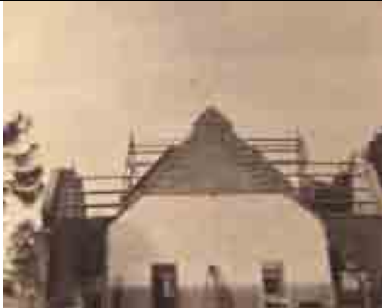
Figure 10.26: Demolition of the Ashby Methodist Chapel, showing the remains of the rear wall, 1939. Source: P. Holden collection, Geelong Heritage Centre, GRS1034.
