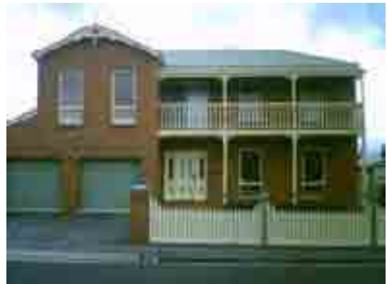
2009: Replacement dwelling, Albert Street.
