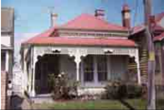
Figure 10.52: "Tragowel", 9 Candover Street, 1986. Source: Aitken, Honman & Huddle, 'City of Geelong West Urban Conservation Study', 1986.
