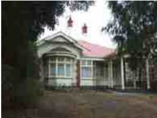
Photo 1: Former Andrews Residence, 230 Latrobe Terrace, Geelong West. Source: David Rowe, March 2009.
