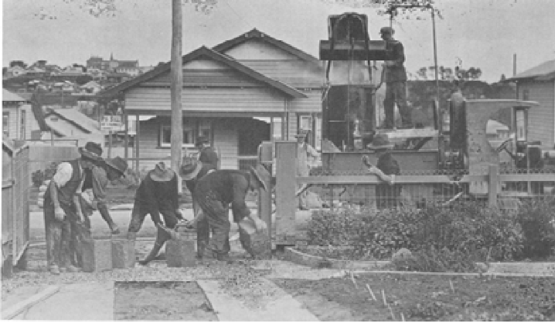
Figure 6.10: Council workers constructing kerbs and channels and footpaths in Geelong West in the 1920s, with the Invicta Road Roller shown in the middle ground. Source: Seaton, The Ashby Story , p.190.
