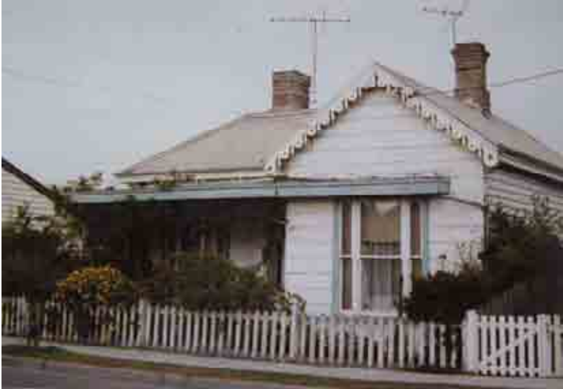
Figure 6.06: "Galloway", 201 Autumn Street, built c.1890. Source: Honman, Huddle & Aitken, 'City of Geelong West Urban Conservation Study', 1986.
