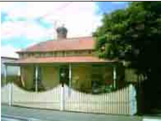
Photo 6.11: Late Victorian dwelling, 57A French Street. Source: David Rowe, 2009.
