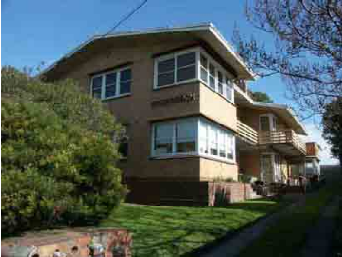
Former Residence, 240 Latrobe Terrace, Geelong West, 2001
