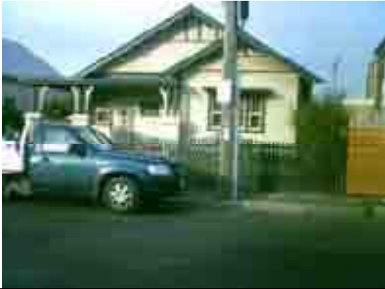
Photo 10.41: Residence, 25 Waterloo Street. Source: City of Greater Geelong, 2008.
