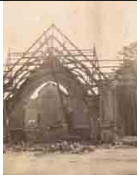
Figure 10.27: Demolition of the Ashby Methodist Chapel from the front (Wellington Street), 1939. Source: P. Holden collection, Geelong Heritage Centre, GRS1034.
