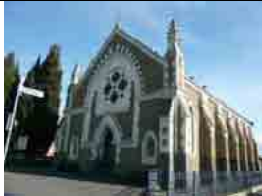
Photo 9.14: Pakington Street Reformed (former Methodist) Church. Source: David Rowe, 2008.
