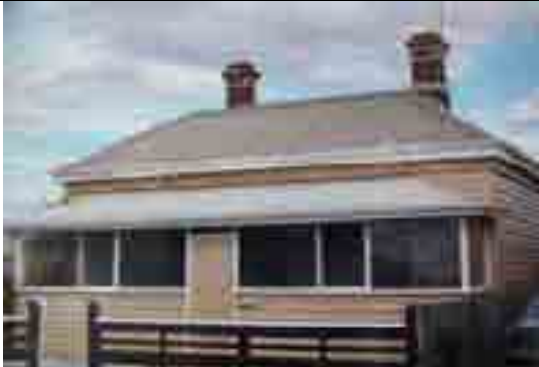
1986: Victorian dwelling, Weller Street, with introduced infill glazing and weatherboards to front verandah.
