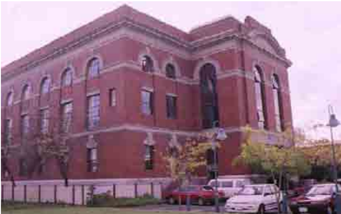
Figure 8: Former Fitzroy North Electric Railway Substation, built in 1915. Source: Victorian Heritage Database online.
