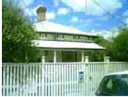
Photo 6.26: Capped timber picket fence to Late Victorian/Edwardian dwelling at 51 French Street. Source: City of Greater Geelong, 2008.
