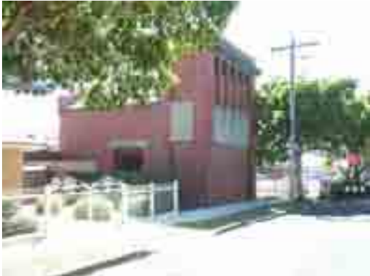
Photo 1: Former electric substation, south and west elevations. Source: David Rowe, January 2009.
