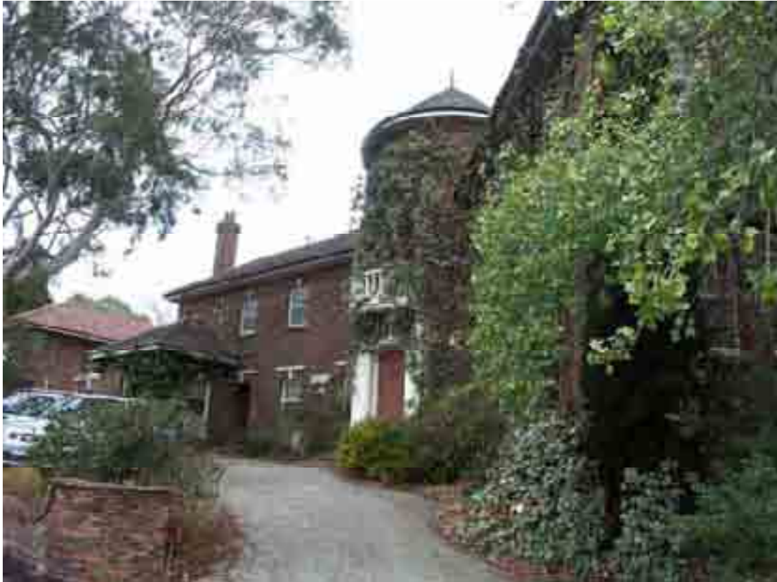
'Narbethong', 242 Latrobe Terrace, Geelong West, March 2009
