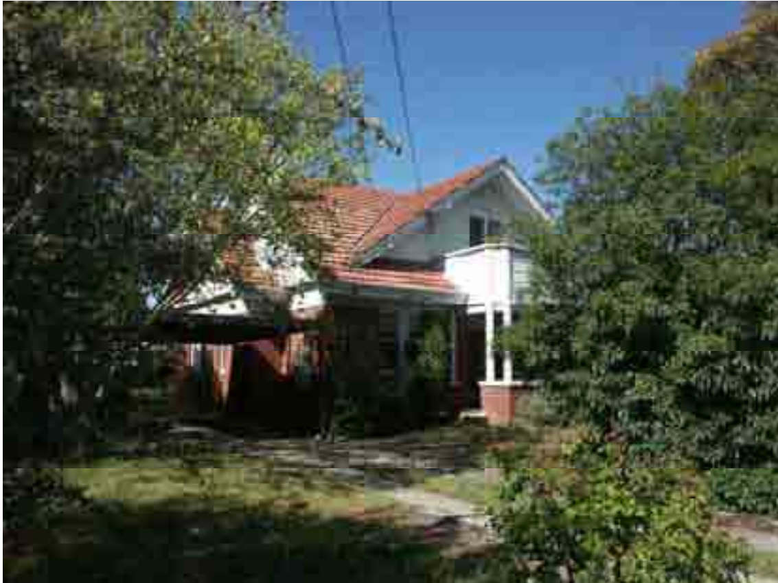
Former St. John's Anglican Church Vicarage, 121 Albert Street, Geelong West, 2009.
