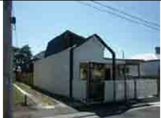
2009: Front contemporary dwelling, with former shed at rear converted to dwelling, Wellington Street.
