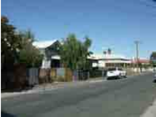
Photo 8.07: Catherine Street, showing Late Victorian and Edwardian dwellings. Source: David Rowe, 2009.
