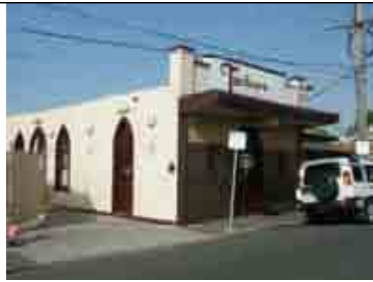
Photo 10.60: Tuckers Funerals building, 57 Hope Street. Source: David Rowe, 2009.
