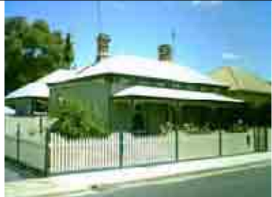
2009: Victorian dwelling, Weller Street, with reconstructed front verandah.
