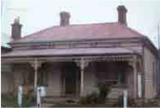
Figure 10.35: “Jersey Villa”, 42 Maitland Street, 1986. Source: Aitken, Honman & Huddle, ‘City of Geelong West Urban Conservation Study’, 1986.
