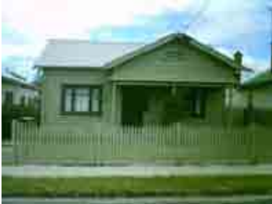
Photo 6.19: Interwar Californian Bungalow, 17 Crofton Street. Source: City of Greater Geelong, 2008.
