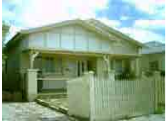
2009: Interwar Bungalow, Ann Street, with introduced timber picket fence.
