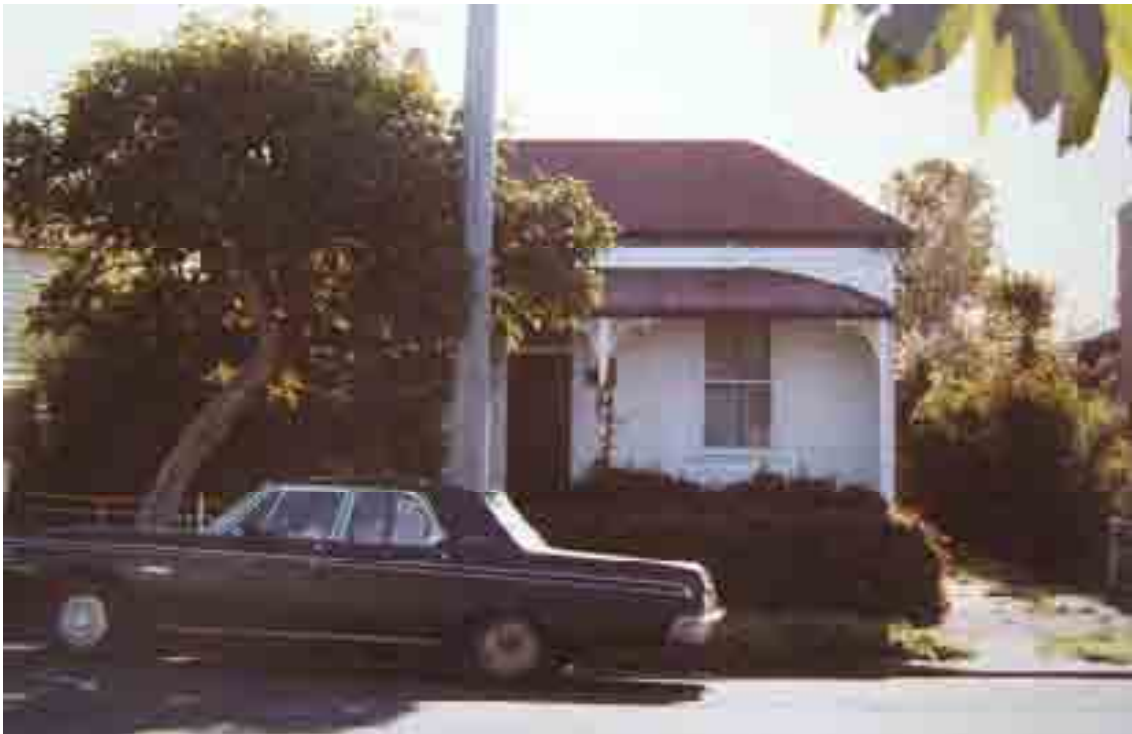
Figure 8.31: Dwelling at 8 Waratah Street. Source: Honman, Huddle & Aitken, 'City of Geelong West Urban Conservation Study', 1986.
