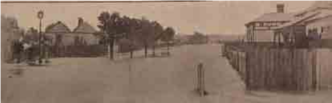
Figure 9.30: Gertrude Street looking west from the intersection with Thomas Street, showing floodwaters from the nearby open drain (West Gully) in 1911. The Late Victorian dwellings at 68-74 Gertrude Street are shown on the right, with the dwelling at 77 Gertrude Street shown in the middle ground on the left. Source: News of the Week , 16 March 1911, Geelong Heritage Centre.
