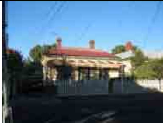
Photo 10.28: Residence, 31 Wellington Street. Source: City of Greater Geelong, 2008.
