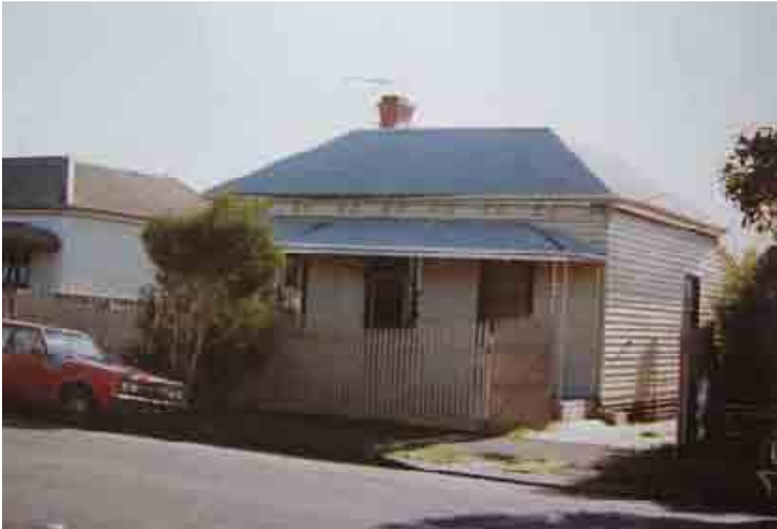
Figure 8.32: Dwelling at 10 Waratah Street. Source: Honman, Huddle & Aitken, 'City of Geelong West Urban Conservation Study', 1986.
