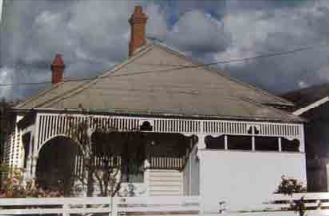
Figure 8.28: “Ivanhoe” at 179 Hope Street, built in 1905-06. Source: Honman, Huddle & Aitken, ‘City of Geelong West Urban Conservation Study’, 1986. The infill to the front verandah has been introduced.
