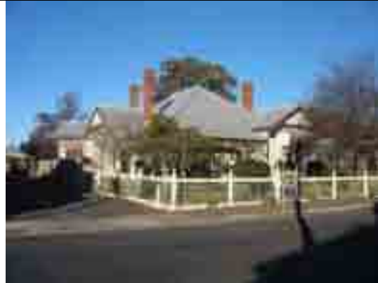
Photo 10.56: "Armagh", 27 Wellington Street. Source: David Rowe, 2008.
