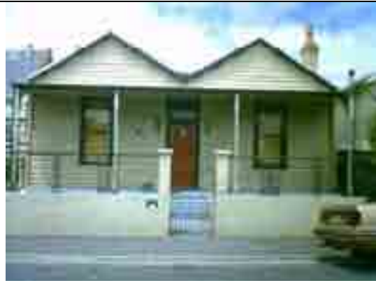
Photo 9.04: Residence, 1 Pizer Street. Source: Pam Jennings, 2008.
