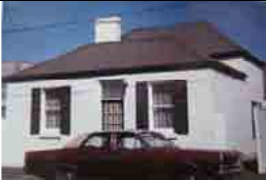
Figure 10.18: Residence, 11 Preston Street, 1986. Source: Aitken, Honman & Huddle, 'City of Geelong West Urban Conservation Study', 1986.
