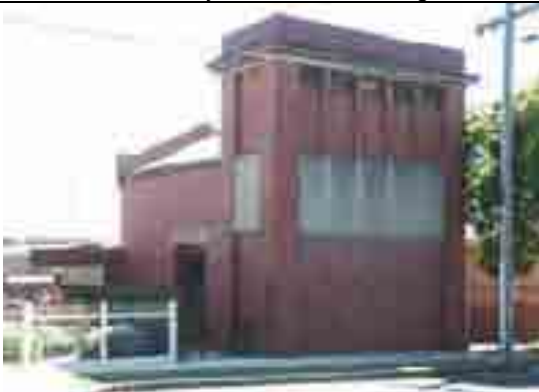
Photo 8.21: Former Substation building to Donaghy's Ropeworks, 2 Waratah Street. Source: David Rowe, 2009.
