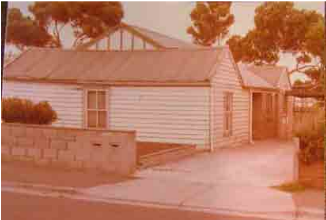
Figure 8.03: Former Baker family residence, 82 Waratah Street, initially built in the 1850s. Source: GRS1160, Geelong Heritage Centre, c.1981-85.
