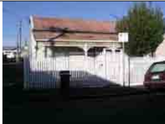
Photo 10.22: Residence, 1 Weller Street. Source: City of Greater Geelong, 2008.
