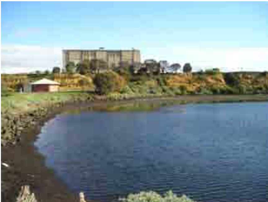
View looking west to the existing cliff face, access ramp and former Powerhouse building
